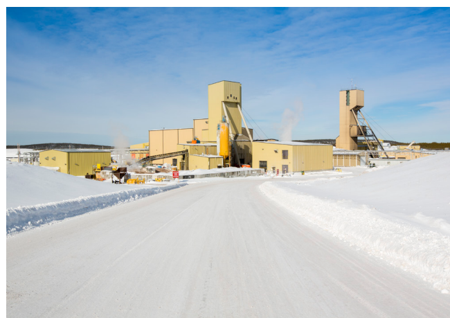
Cigar Lake-mijnsite in Canada (foto: Cameco Corporation)
