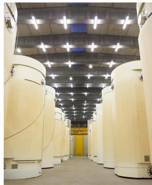
Dry storage casks at the Doel nuclear power plant (Electrabel photo library)
