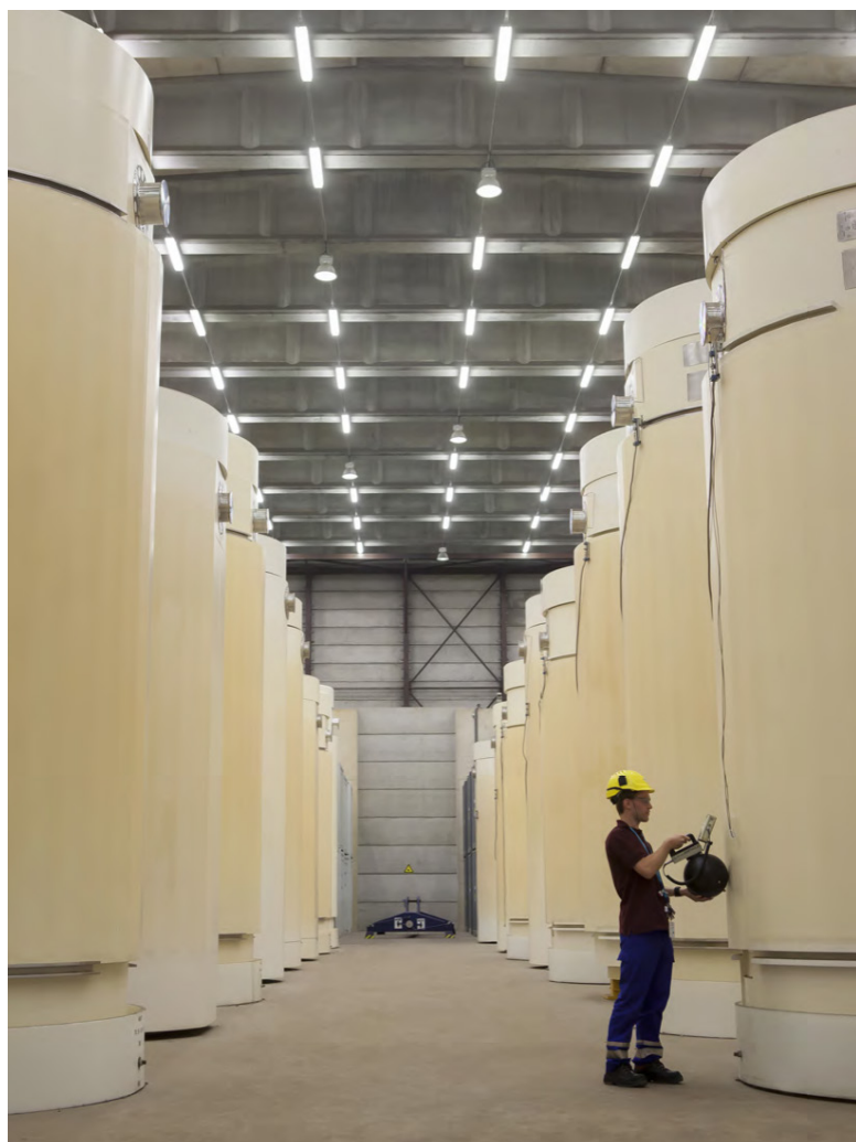
Doel nuclear power plant. Centralized building housing dry storage casks for spent fuel. ELECTRABEL Photo Library
